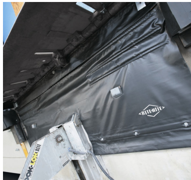
PitMaster Under-leveler Seal.
