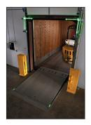
Corner-Vu and Leveler-Vu, part of the Rite-Vu<sup>™</sup> Light Communication System, enhance visual communication of the Dok-Lok control box.
